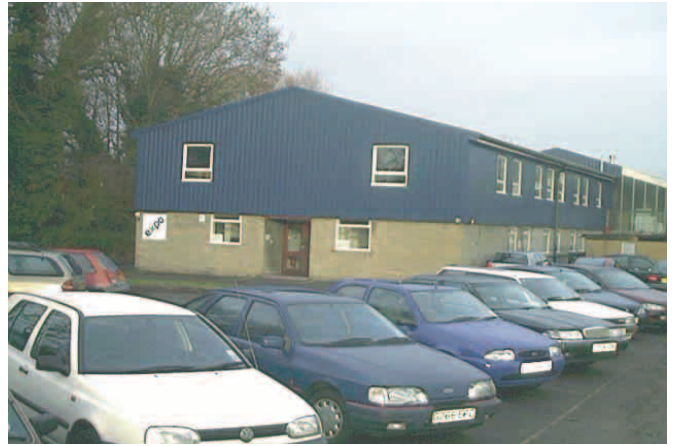
Expo Technologies main engineering and manufacturing facility
